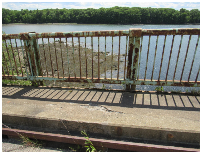
Typical Existing Bridge Rail Section
