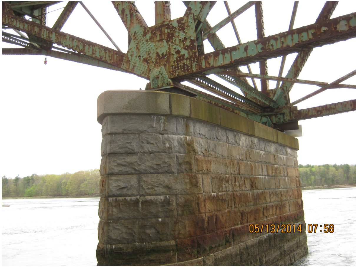
Pier 4 Node Looking Upstream
